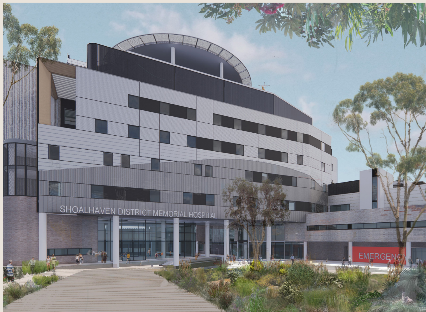
Render of new Shoalhaven Hospital entrance. Image: supplied
